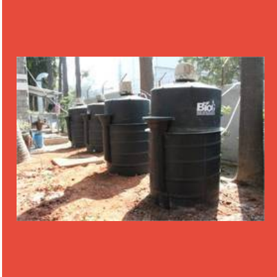
Biogas Plant (Domestic)
